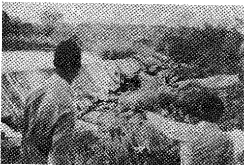
Figure 3. Concrete dam construction (Mumbwa)
