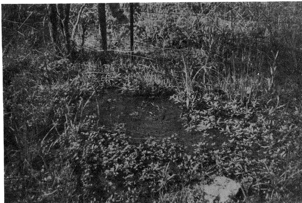
Figure 9. Leakage of a raw water main.
