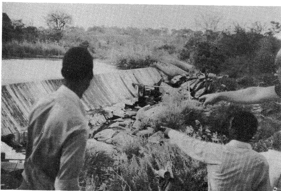
Figure 3. Concrete dam construction (Mumbwa)
