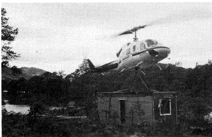
Fig. 9. The barracks were transported from a nearby road by helicopter
