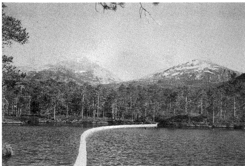
Fig.2. A plastic curtain divides the Lake into two separate basins
