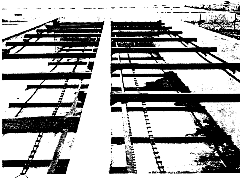
Figure 5.2 Rectangular primary sedimentation tank with wood flights mounted on parallel chains.
