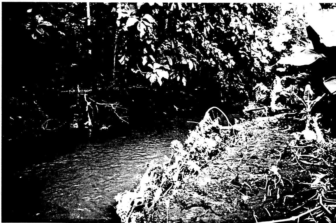
Figure 4: The old treatment plant in Moshi, with overgrown ponds and outlet of sewage to Njoro river.
