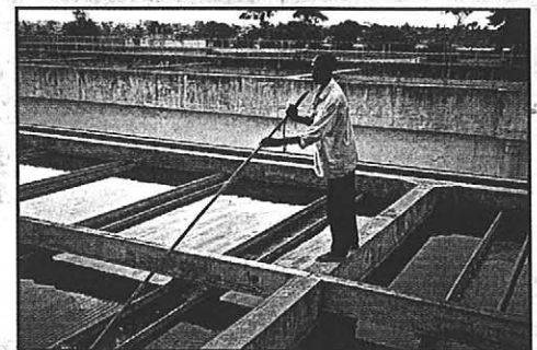
Water treatment plant maintenance
