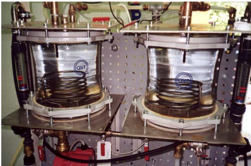
Figure 4. Hot water tanks after cleaning with acid
