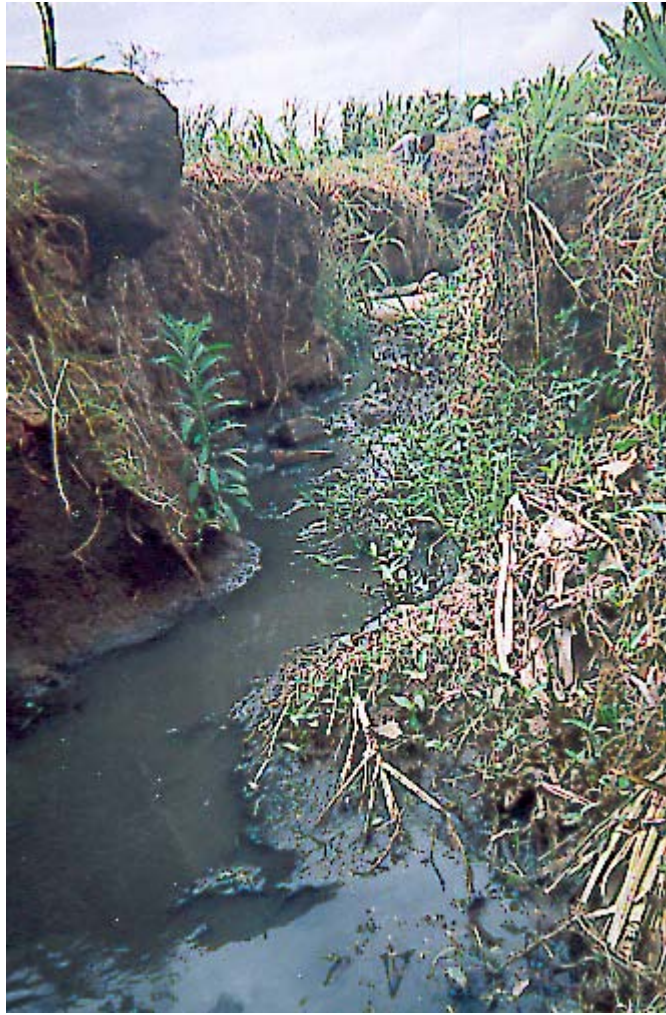
B.5 Sewage stream from broken pipeline
