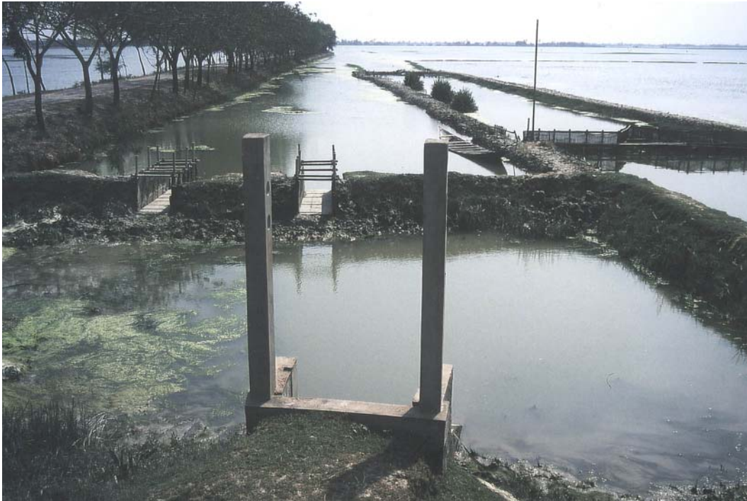
Figure 2 Main water inlet at Soladana shrimp farm
