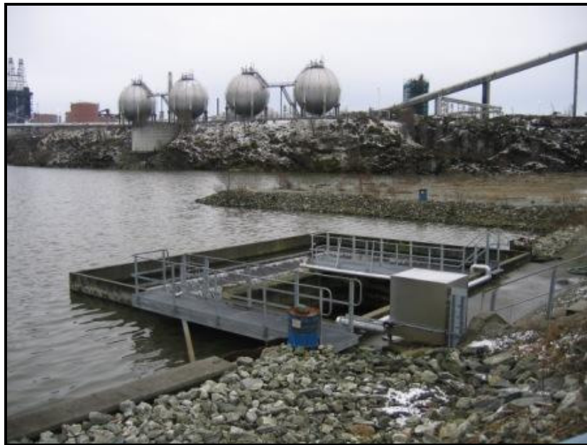
Figure 6. Photo showing the pit where the discharge pipeline begins. The STD measurements were taken just at the concrete wall, at ca. 80 cm water depth.
