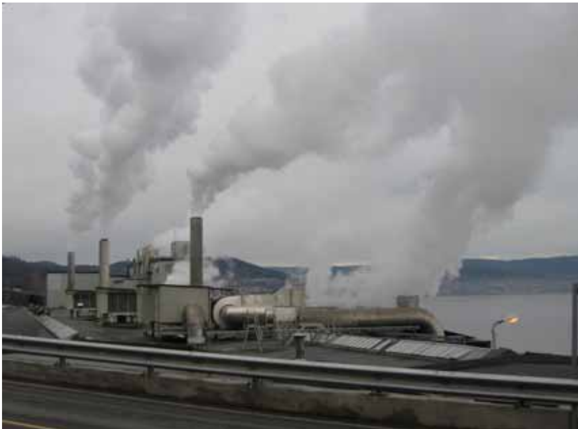
The plant of Norgips Norge AS at Tørkop Photo: Jarl Eivind Løvik
