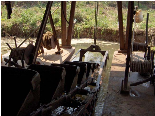
3. A continuous excavator belt with half a meter between the grabs is fairly efficient.
