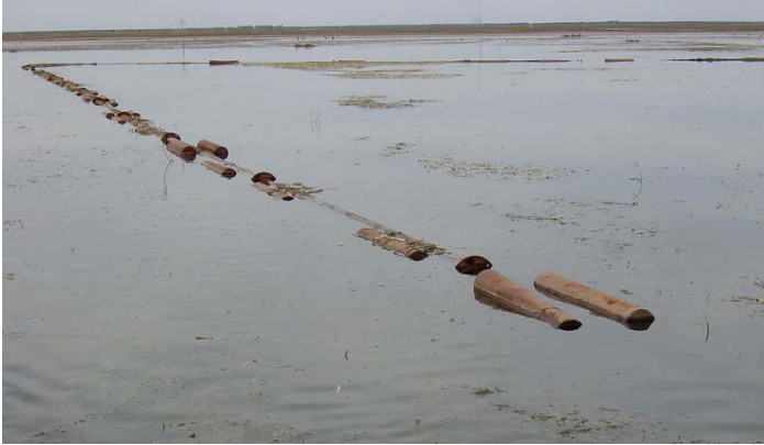
Figure 3.6 Pipe-line transports the excavated material to the shore
