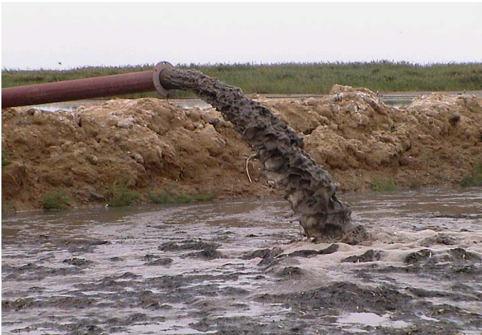
Figure 3.7 Excavated material pumped into the lagoon
