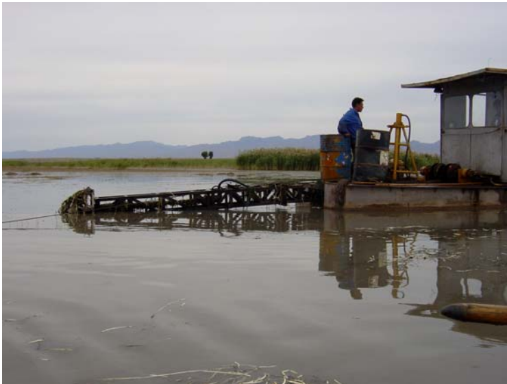
Figure 3.4. Dredging barge in action on lake Wuliangsu Hai
