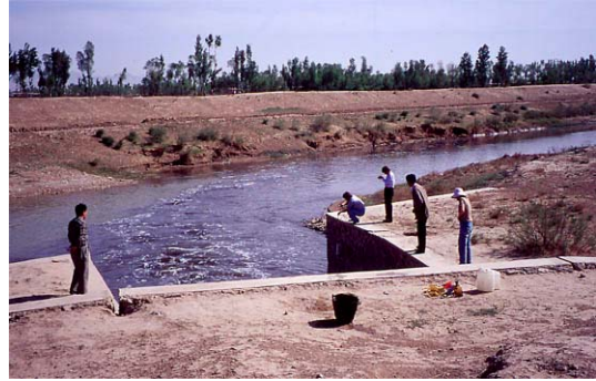
Drainage canal no. 3
