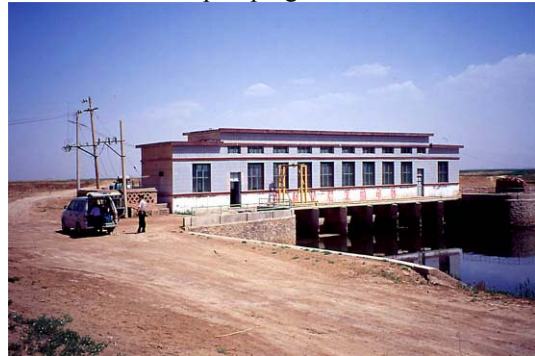
Drainage canal no. 9 At pumping station
