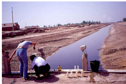
Drainage canal no. 7
