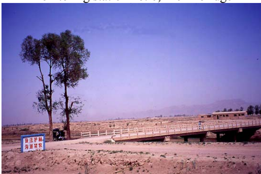
Main drainage canal, monitoring station no. 6, Melin bridge
