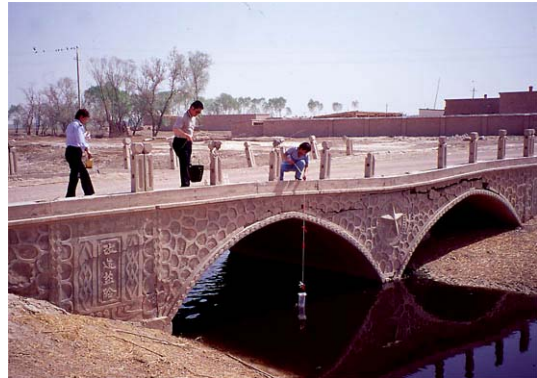
Drainage canal no. 5
