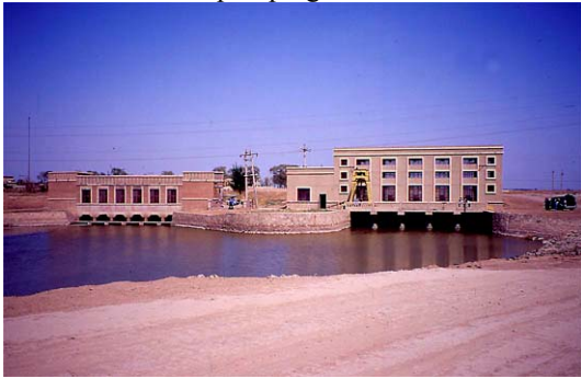
Drainage canal no. 8 At pumping station
