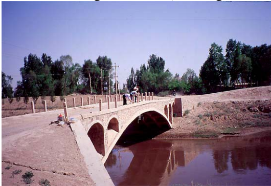
Main drainage canal, monitoring station no. 4, Yindingtu
