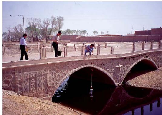
Drainage canal no. 5
