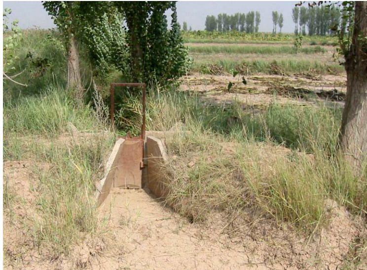
Figure 4.8 Typical gate for regulating water flow into the farmland. Photo: Hans Ljungquist, Global School
