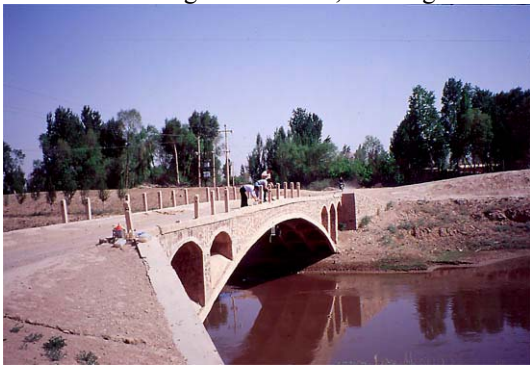
Main drainage canal, monitoring station no. 4, Yindingtu
