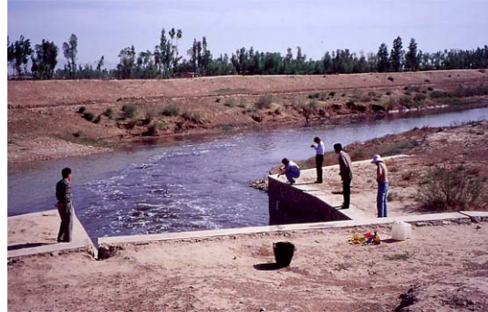
Drainage canal no. 3
