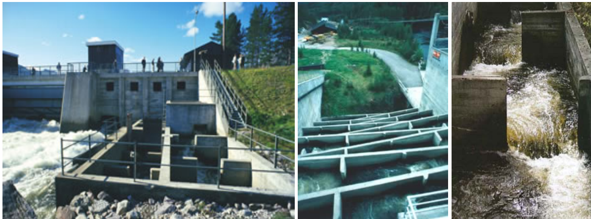
Figure 14-1. Left panel: Høyegga Dam with fish ladder, Centre: The fish ladder at Løpet Dam (both Glomma River). Right: Close-up of the fish ladder canal. Photo: Left and centre: GLB, right: Tore Qvenild 2008.
