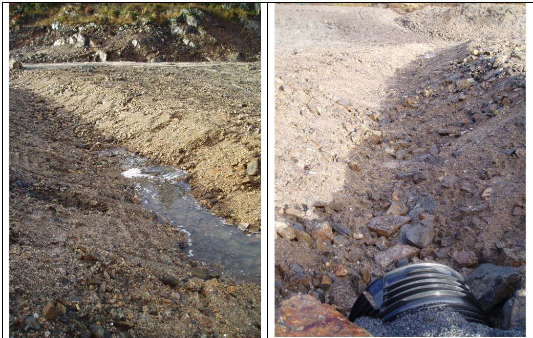
Figure 15. Open ditch across M17 on November 17, 2009. The stream in the picture to the left was supposed to cross the fill and enter the pipe in the picture to the right. Instead, it runs into the fill halfway over.
