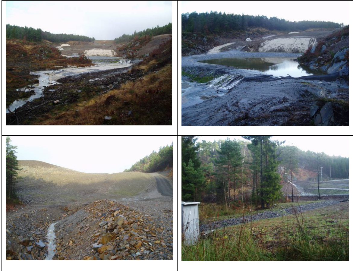
Figure 2. Deposit M17 (upper panel) with fill area, lower dam and downstream area with shell sand and gravel on November 17, 2009. Sampling point was at the dam outlet and 200 m downstream, at the base of the picture to the left. Deposit M20 (lower panel) with fill area, and outlet stream on November 17, 2009. The yellow-brown colour of the sulphide-bearing rock is clearly seen. Picture to the right shows the pH-measuring and sampling point 200 m downstream.
