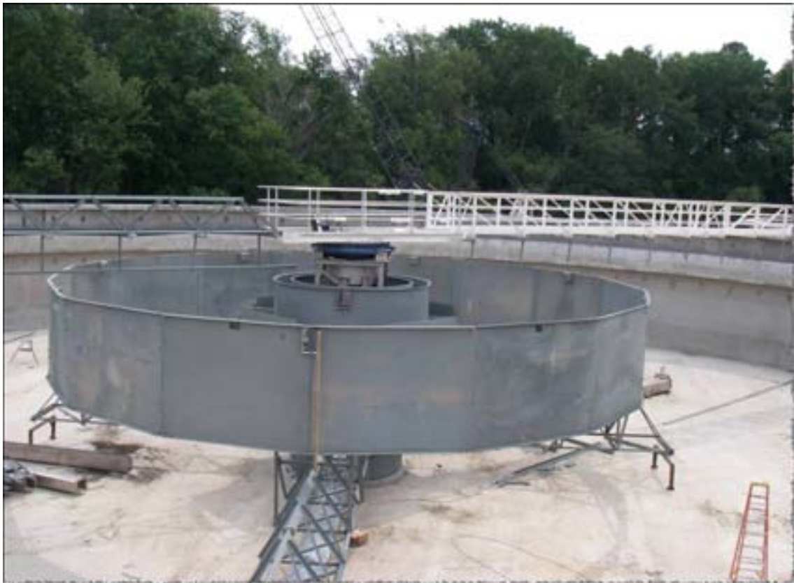
Figure 15. Structure of a secondary clarifier ( http://www.hrsd.state.va.us/images/ATP/Secondary%20Clarifier%20Equipment.jpg )
