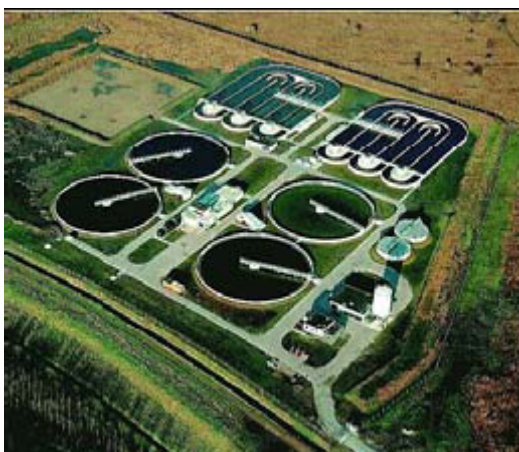
Figure 10. Carrousel oxidation ditch process developed by DHV ( http://water.dhv.com/NL/waterbehandeling/afvalwater/Documents/Leaflet_Carrousel.pdf )
