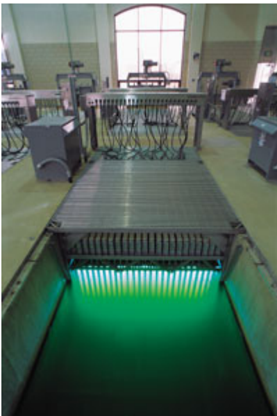
Figure 17. UV disinfection of wastewater effluent ( http://www.mindfully.org/Water/UV-Disinfection-Wastewater.jpg )
