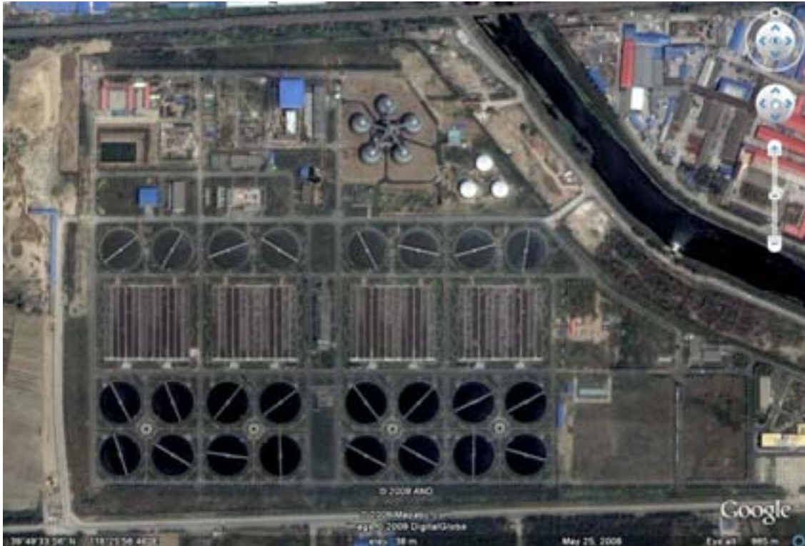
The overall layout of the plant
