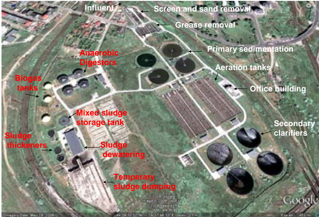
Figure 45. Constanta South Wastewater Treatment Plant (4 units of anaerobic digestors and three biogas tanks are used today)
