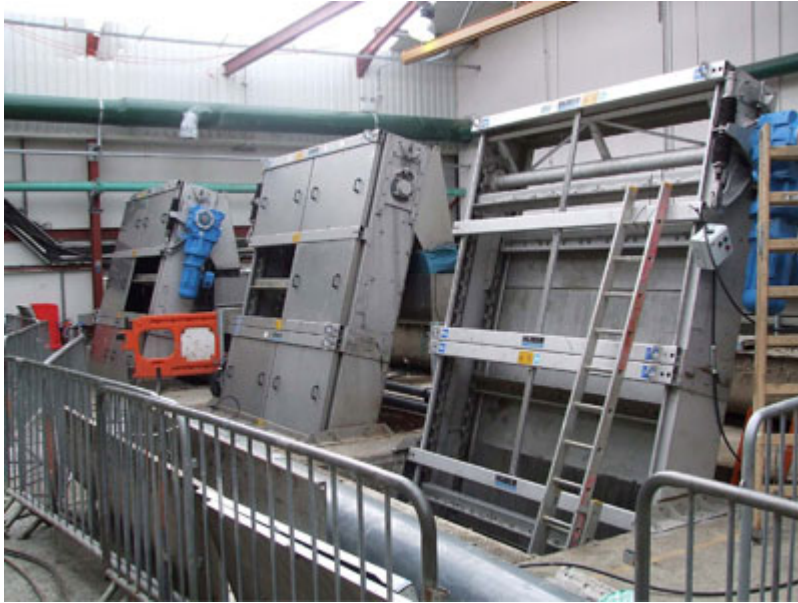
Figure 5. Coarse screen for removal of bigger particles
