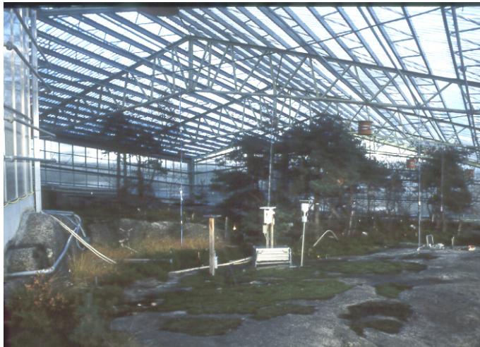
Risdalsheia in Norway – a 1200-m 2 roof removing the acidic input to a complete catchment. Effects on plants, soil and water were studied (Wright et al. 1993).
