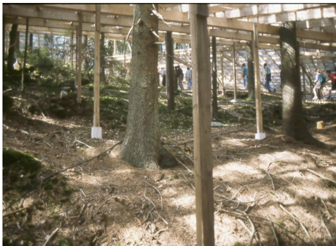
Gårdsjön in Sweden – a 7000-m 2 roof built underneath the forest canopy of a complete catchment to remove the acidic input to the soil and replace it with clean rain (Hultberg and Skeffington 1998).
