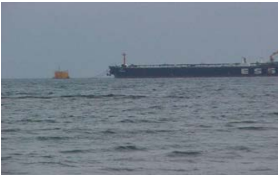
Figure 76: The Single Point Mooring (SPM) system used for loading oil tankers at the Bashayer marine oil terminal. The SPM is located approximately 2 km off the coastline.
