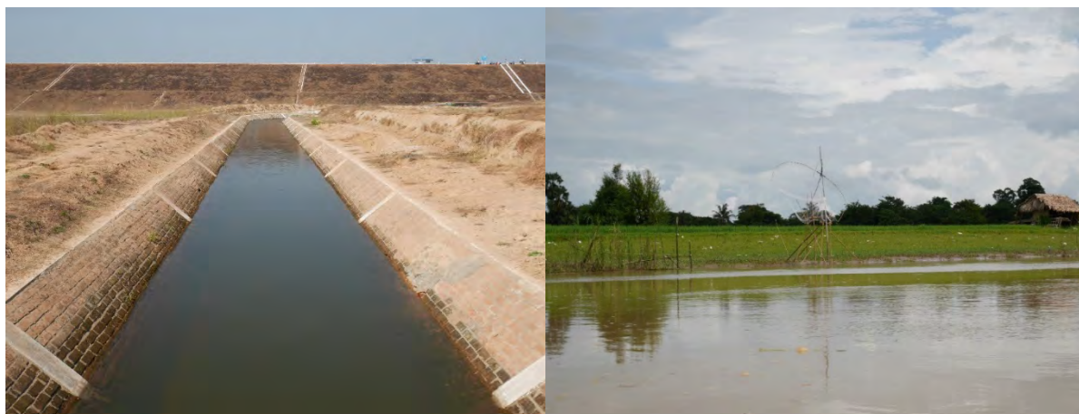
Figure 3.4 Embankments made to the Mazin Chaung in upper parts (upper) and the Eastern bank of the Bago River Between the Bago City and Tawa Village (lower).
