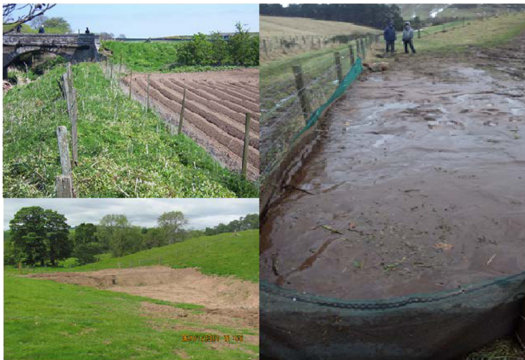
Fig. 1. Clockwise from top left (a) 2 m regulatory buffer strip for protection of water course from sediment runoff from adjacent potato field, which also shows infield measure of contour furrows on end rig of the field (b) targeted sediment fence constructed in Dec 2014 at margin of field in aftermath of Brussels sprouts (c) detention bund constructed at base of gully running through field currently in grass. The site was chosen as high risk after large erosion losses after the field was in potatoes.
