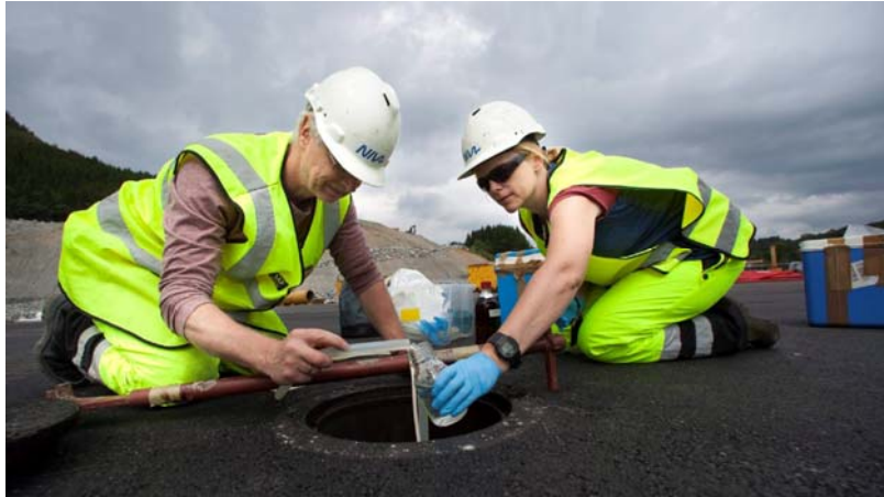
Figure 10: Groundwater samples from four wells in the quay deck are collected for analysis of contaminant levels.
