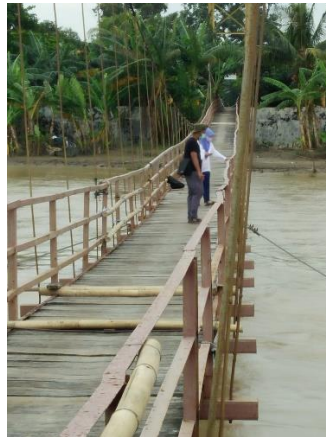
Figure 4. Observation using visual counting on the bridge.
