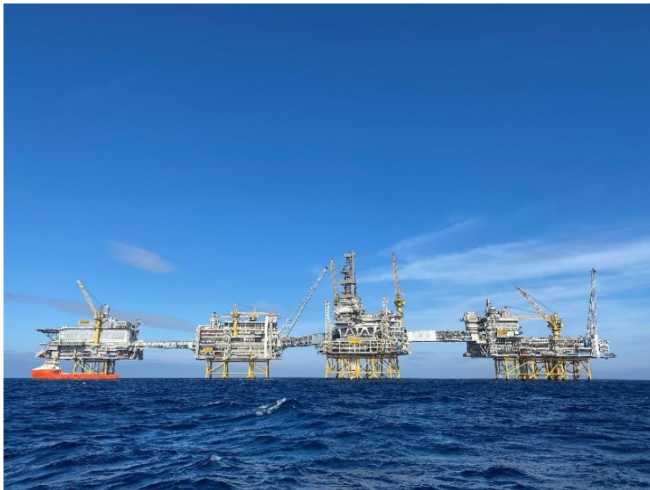
Figure 1. The Johan Sverdrup complex comprising from left to right of the accommodation platform, the process platform, the drilling platform and the riser platform. (Source: Steven Brooks, NIVA).
