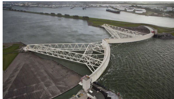
Figure 10. Example of a storm surge barrier. Source: Delta Works | Rijkswaterstaat.
