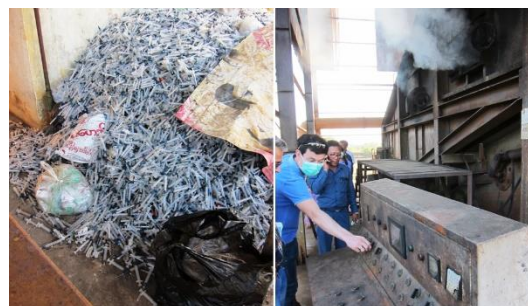
Syringes and sharps incinerated in an old incinerator operated by MDCDC in Mandalay without any flue gas treatment (Photo: SINTEF)
