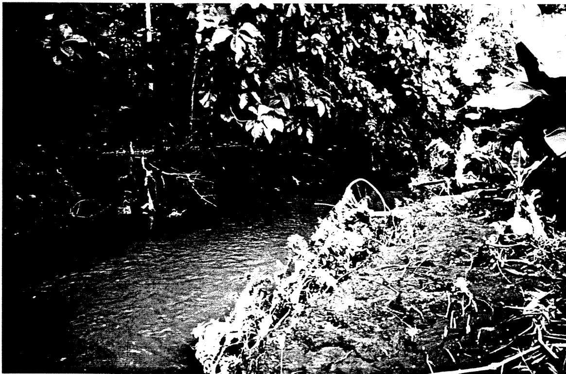
Figure 4: The old treatment plant in Moshi, with overgrown ponds and outlet of sewage to Njoro river.
