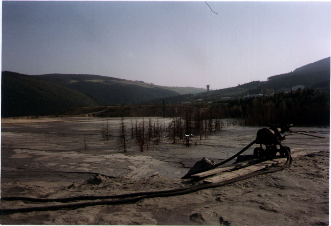
Figure 2 Tailings pond 03 in operation at Zlaté Hory-South (April 1992).
