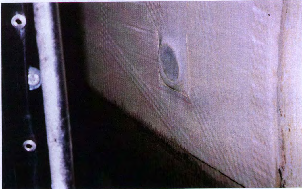
Photo 1 Filter plate after flushing the feed pipeline into the press.
