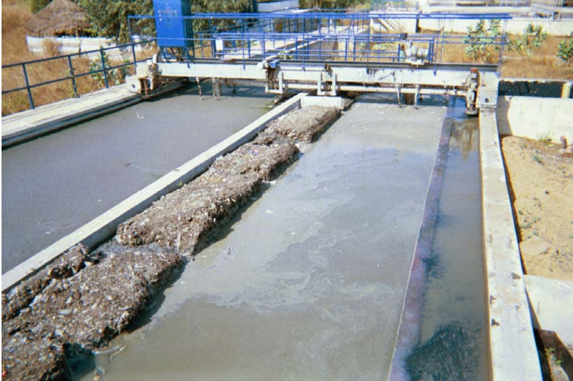
Figure 4. Grid chamber of Cambérène Sewage Treatment Plan
