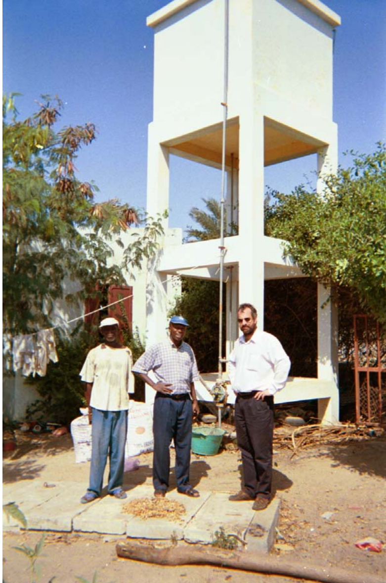
Figure 5. Overhead tank in Rufisque
