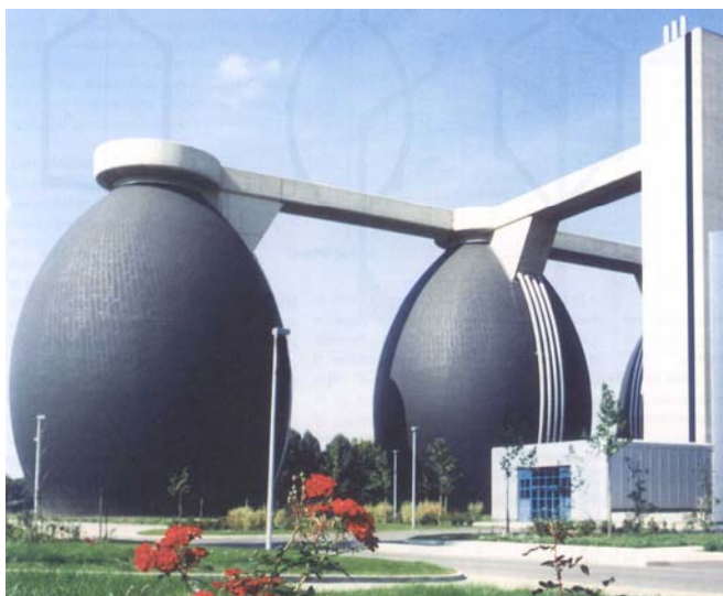
Figure 77. A modern anaerobic digester
