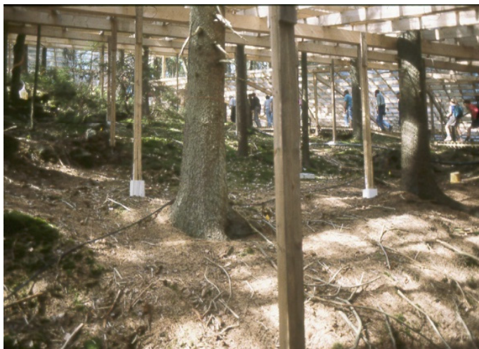
Gårdsjön in Sweden – a 7000-m 2 roof built underneath the forest canopy of a complete catchment to remove the acidic input to the soil and replace it with clean rain (Hultberg and Skeffington 1998).
