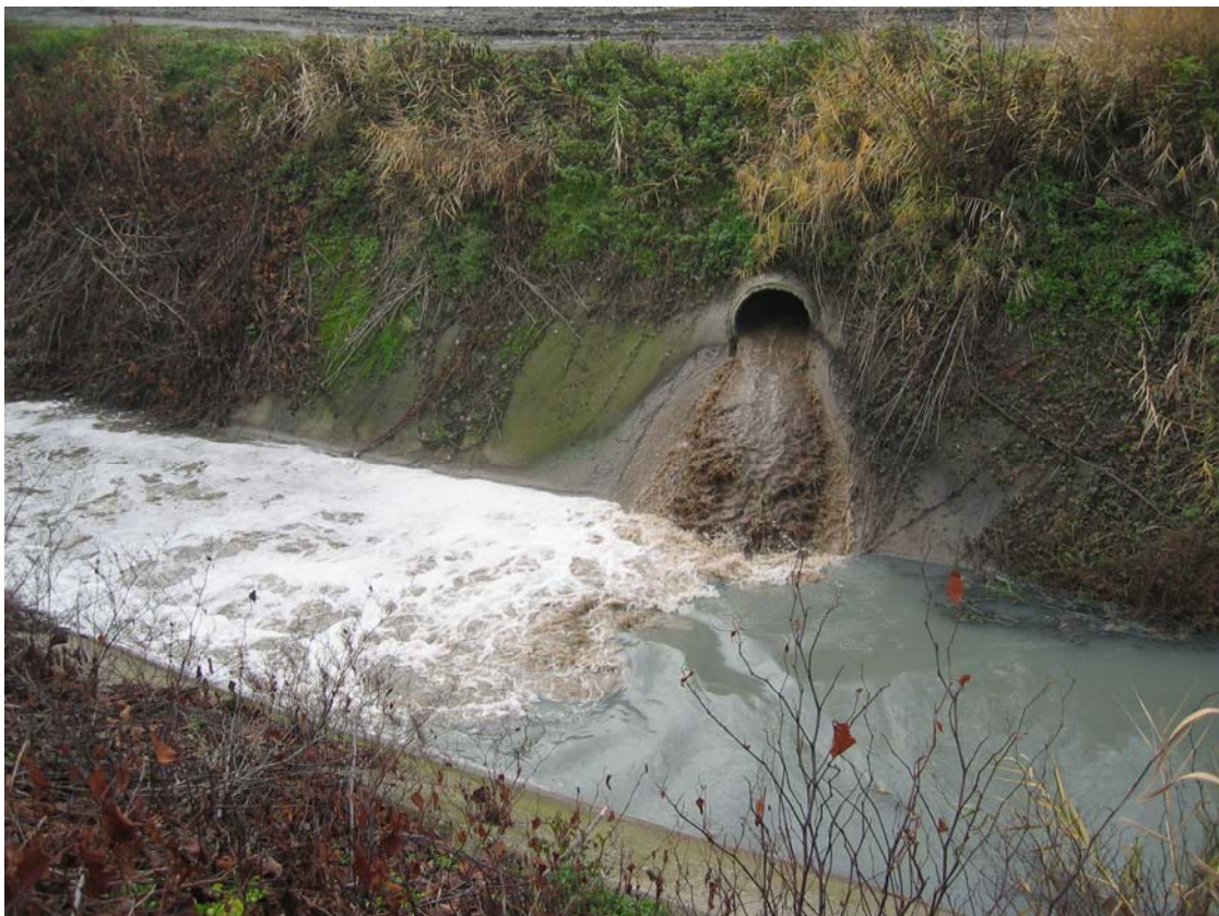
Industrial effluents are discharged untreated via I-64 lateral into the DTD-Canal
