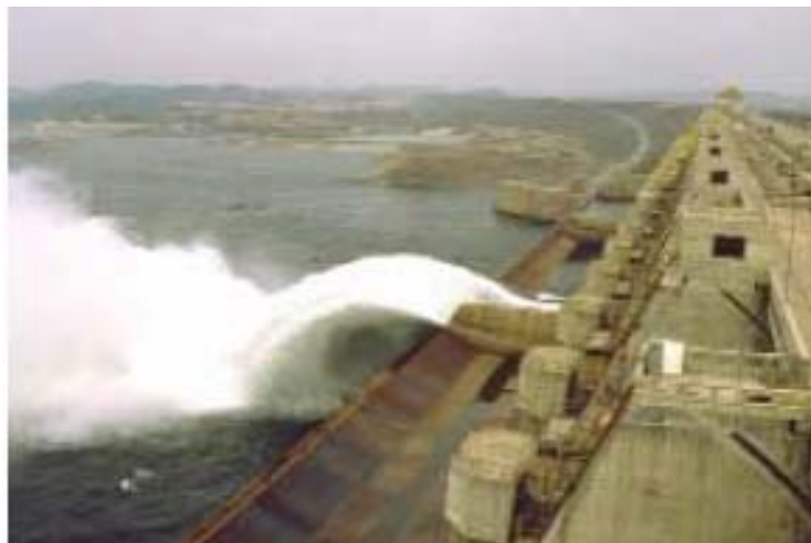
Figure 26. Hypolimnion spillway release in the Tucuruí dam, Brazil (Fearnside 2002). The ski-jump fashioned release of the spillway was constructed to effectively oxygenate the water. But, at the same time it is efficient in stripping off the methane and carbon dioxide content of the reservoir deep water.
