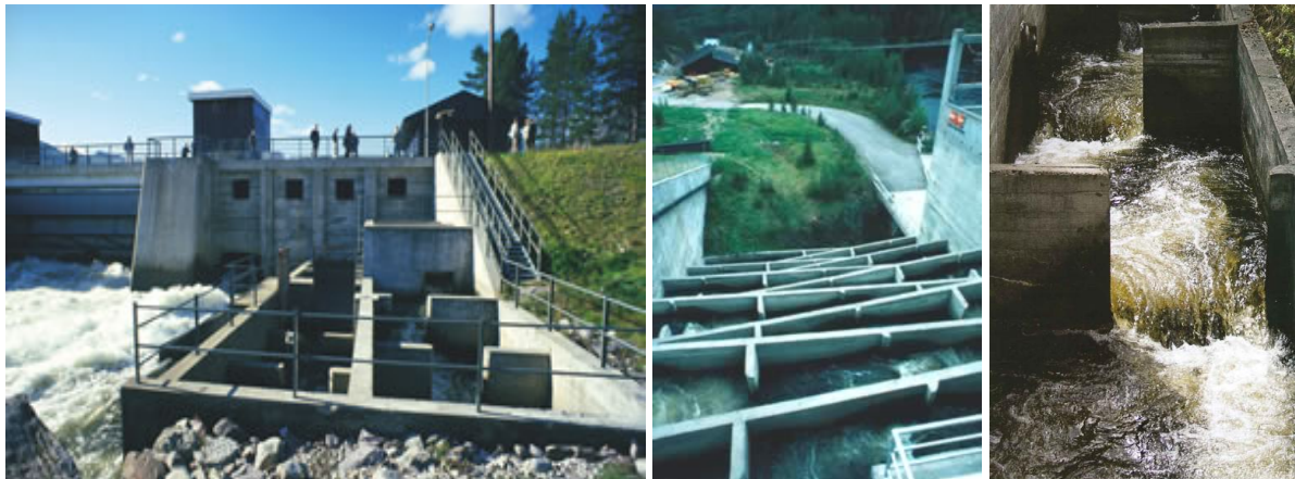
Figure 14-1. Left panel: Høyegga Dam with fish ladder, Centre: The fish ladder at Løpet Dam (both Glomma River). Right: Close-up of the fish ladder canal. Photo: Left and centre: GLB, right: Tore Qvenild 2008.
