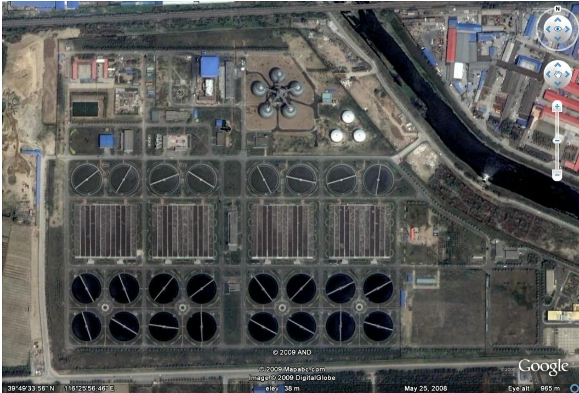
The overall layout of the plant
