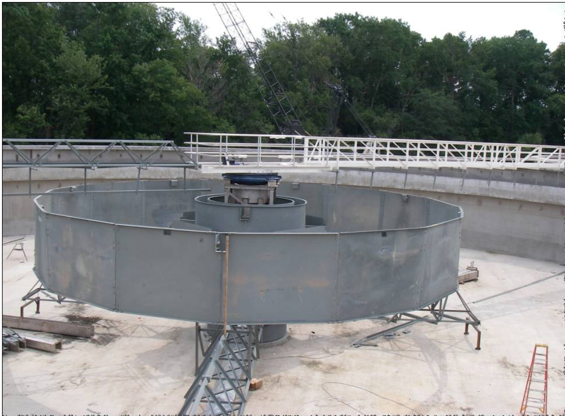
Figure 15. Structure of a secondary clarifier ( http://www.hrsd.state.va.us/images/ATP/Secondary%20Clarifier%20Equipment.jpg )
