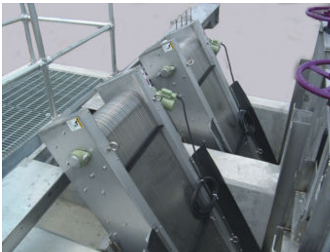
Figure 6. Fine screen for removal of fine particles
