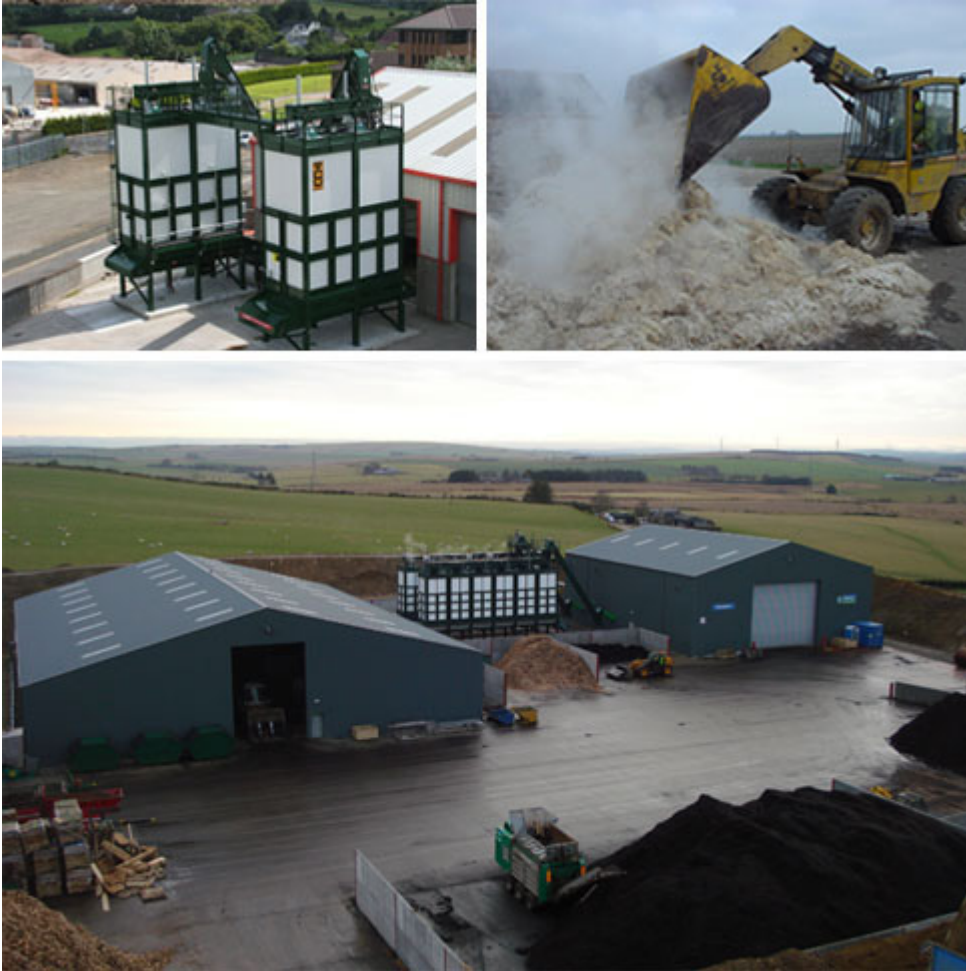
Figure 25. In-vessel composting
