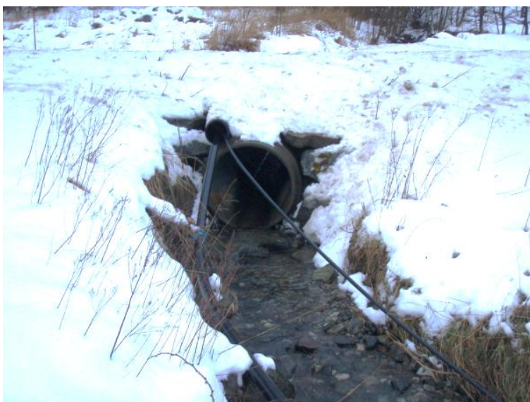
Figur 19. Kulvert under Rv 55.
