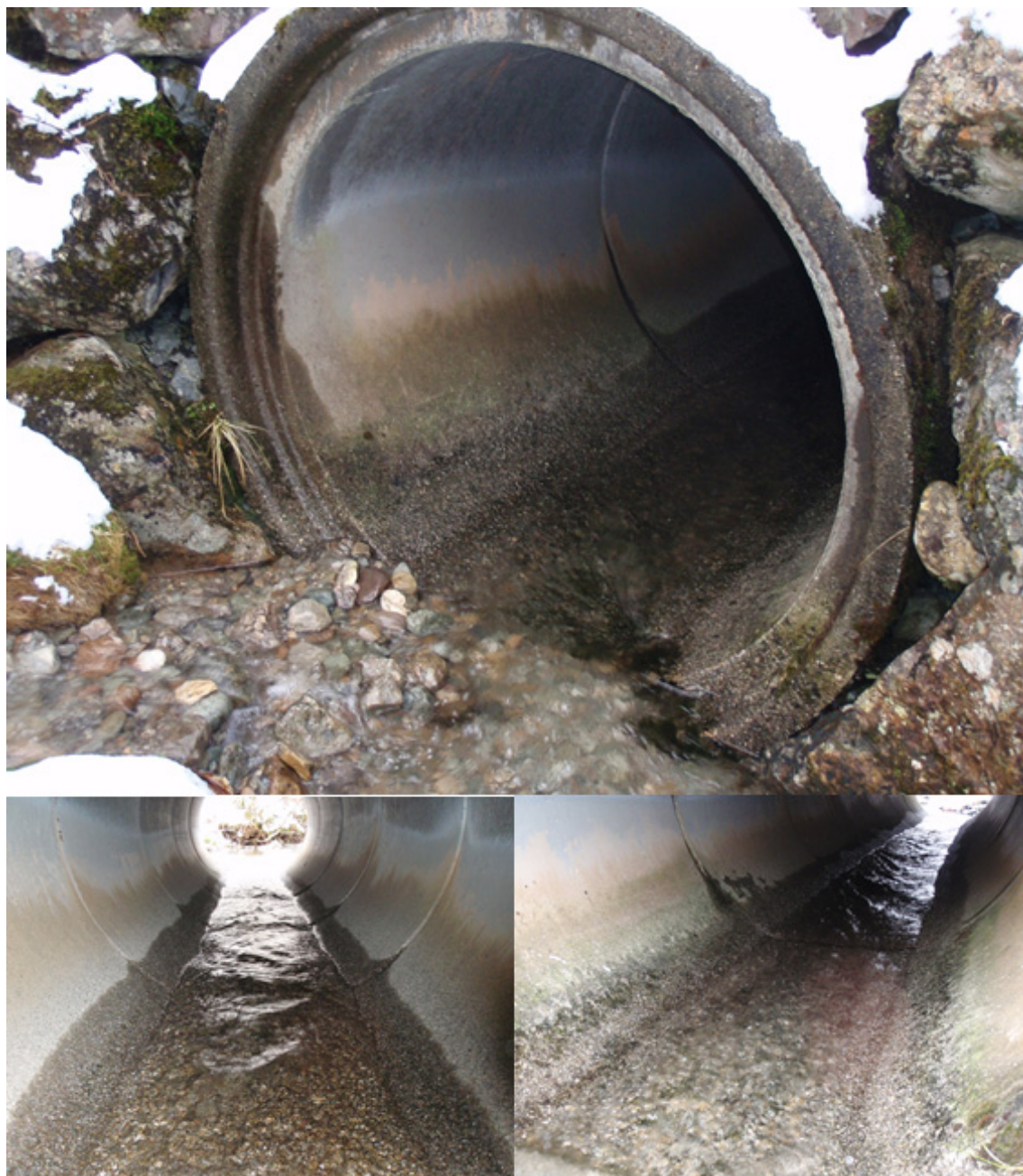
Figur 50. Betongkulvert under 615.
