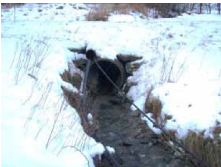
Figur 19. Kulvert under Rv 55.
