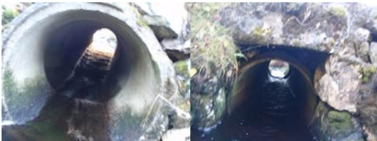
Figur 120. Kulvert under Fv 342.
