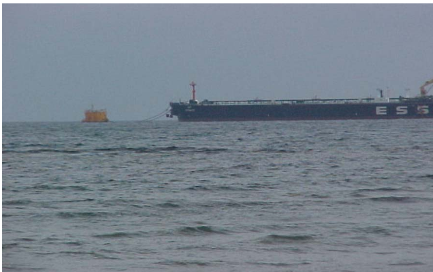
Figure 76: The Single Point Mooring (SPM) system used for loading oil tankers at the Bashayer marine oil terminal. The SPM is located approximately 2 km off the coastline.
