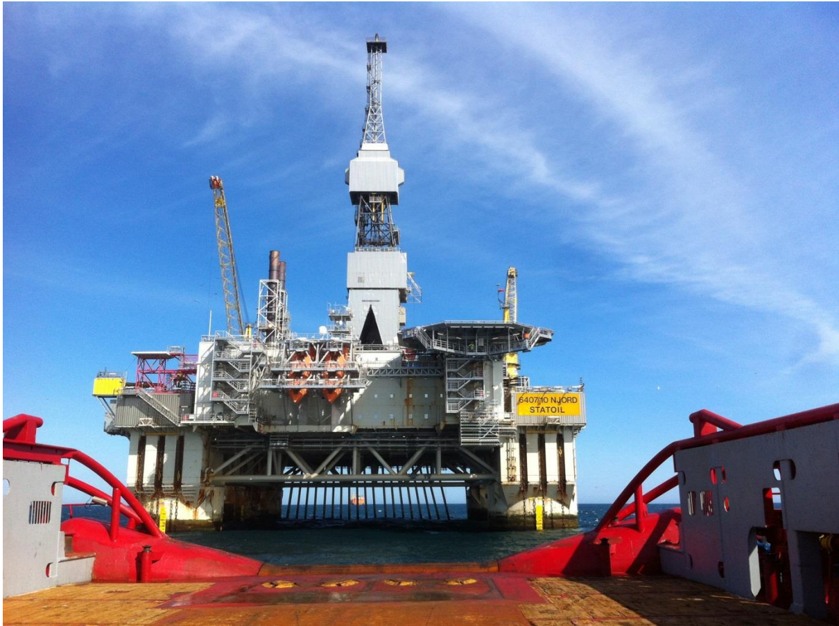
Figure 5. The Njord A platform.
