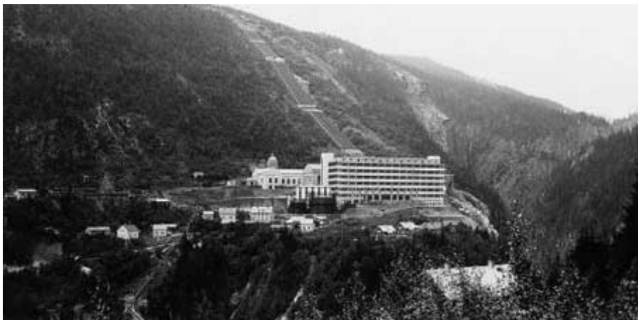
Figure 1. Vemork Power Plant. Norway's first large HP- plant was finished in 1911. Source: reiseliva.wikispaces.com
