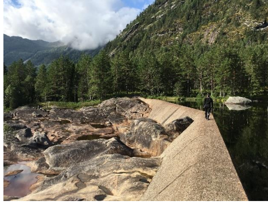
Fig. 18. The site is located right upstream a large weir
