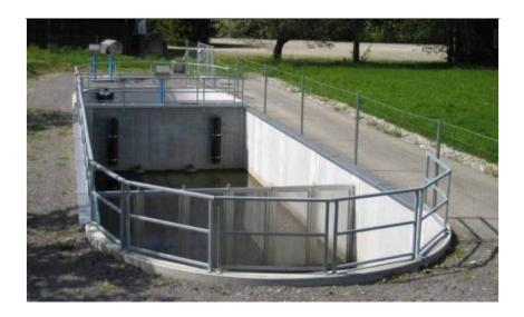
**Figure 6.18 Units based on filtration**: A pre-sedimentation catchbasin (in front) and a down-flow <u>media filter</u> treating first flush (15 min, one-year return period) in Austria (Photo: Courtesy of ASFINAG).
