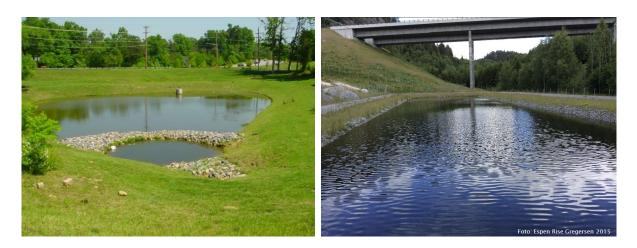
**Figure 5.2** Examples of **wet ponds**. Left: In North Carolina (Photo: City of High Point). Right: Hobekk, E16 in Vestfold (Photo: Espen Rise Gregersen, Statens vegvesen).
