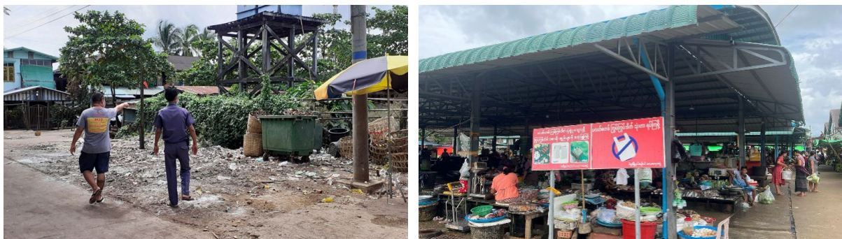
Figure 4.7. Photo (left) shows the area outside of the Phyazay market that was to be restored (August 2020); the photo (right) shows the inside area of the Phyazay market in November 2023 (Source: Kyaw Min San).
